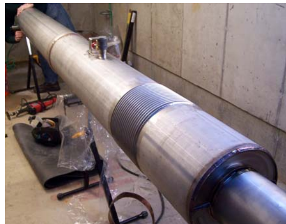
Figure 3: Completed cable joint in vault.
