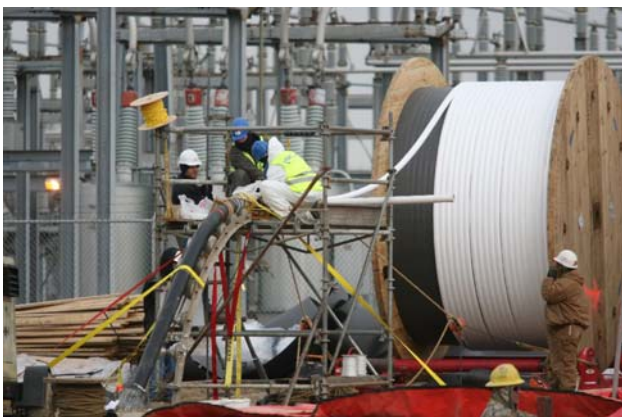
Figure 2: HTS cable installation process.
