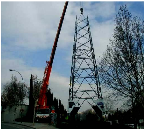
Figure 14: Overhead line dismantling
