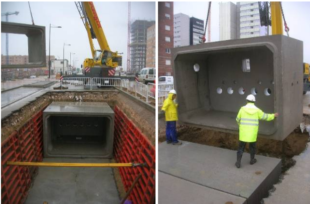
Figure 10: new joint bay
