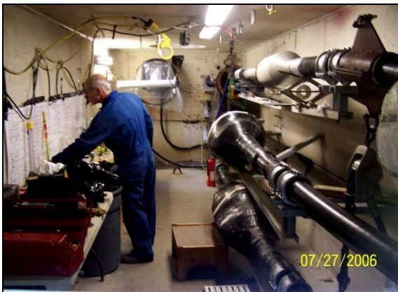
Figure 8: Preparation of splices in manhole
