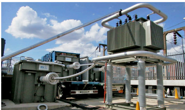
Fig. 6 Mobile AC test system (280kV test voltage)
