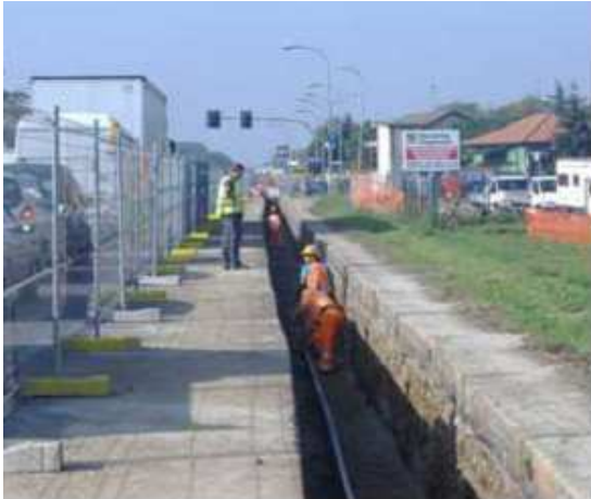
Figure 4: Installation operation along heavy traffic road
