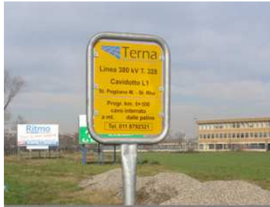
Figure 6: Marking of the cable position along the route.
