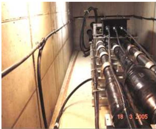
Figure 2: View of the joints manhole
