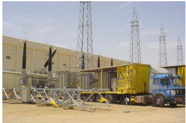
Figure 7: Test of a 380 kV cable in Jeddah / Saudi-Arabia
