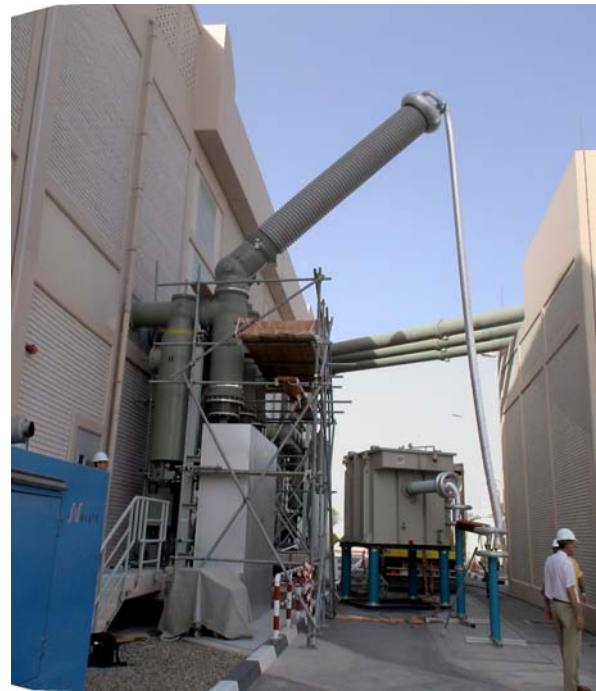
Figure 19 : arrangement for after laying tests at the GIS terminations
