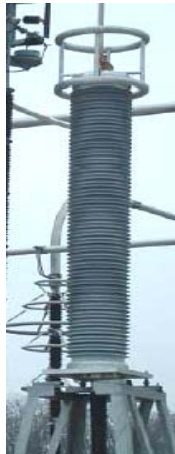
Figure 2 Outdoor composite termination
