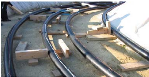
Figure 11 : Controlled backfill area before backfilling
