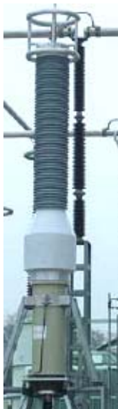
Figure 3 : GIS termination and outdoor bushing
