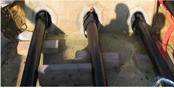
Figure 10 : Ducts area before bentonite® filling
