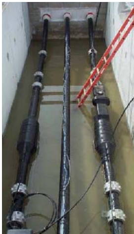
Figure 12 : Joint bay during salted water filling
