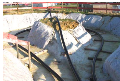
Figure 15 : loop U turn before backfilling
