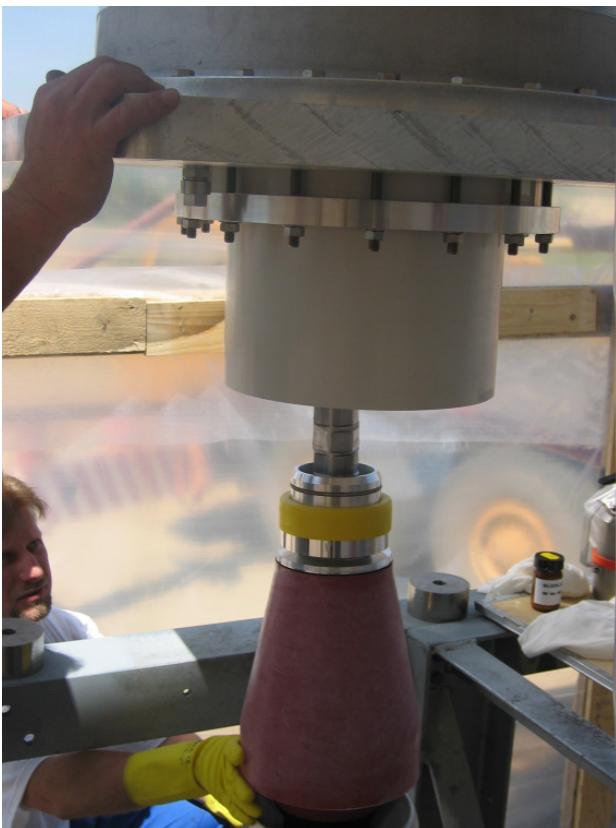
figure 7: installation of bushing part on plug-in part
