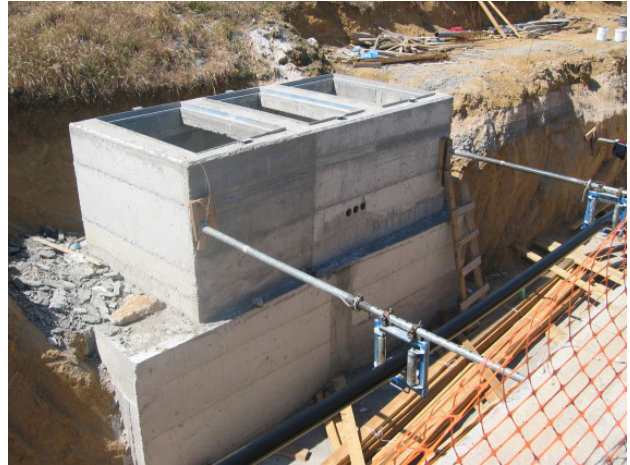
figure 4: joint pit with pre-fabricated concrete elements
