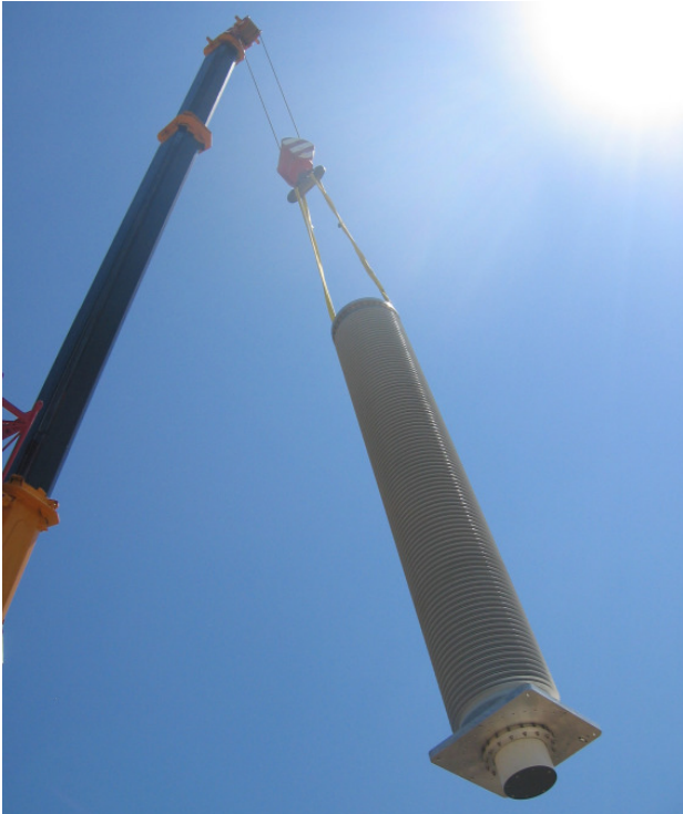
figure 6: moving of pre-fabricated bushing part at job-site
