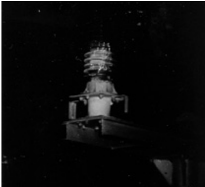
Fig. 1. Discharges on surge arrester
